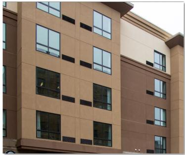
EIFS with Drainage System, is the predominate method of EIFS used today. EIFS with Drainage helps to eliminate moisture before it has an opportunity to enter the wall cavity.
